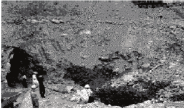
Fig. I-17. Tunel Ching-Gang, Chi-Chi, Tajvan 1999
