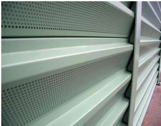
Foto 3.1. (a) Barriera metalike (celik apo alumin)
